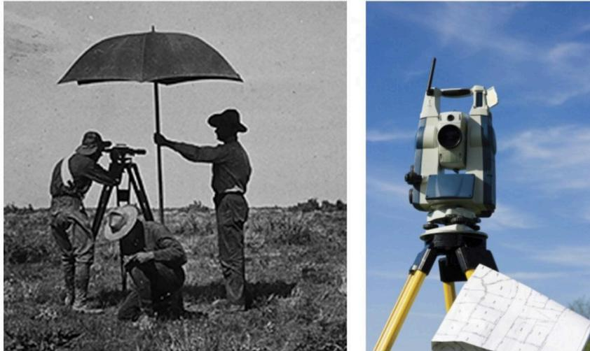
Land surveying. The foundation for modern mapping was laid by people walking and measuring the land with specialized telescopes (left) and modern GPS enabled total stations (right).<sup>23</sup>
